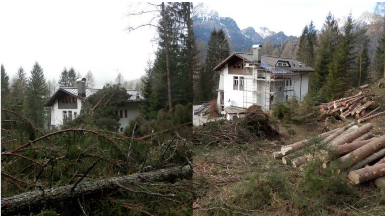
Figure 1. Left: Alpine Ecology Center (Belluno, Dolomites, Italy) on October 30, 2018, on the day after the event. Notice fallen trees on the roof of the building and part of the damages done in its vicinity. Right: Same position two months later (January 4, 2019), with the first restoration works (Photographs: Roberto Menardi).
